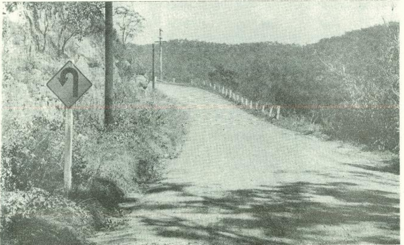
Photograph 6. Settlers Road - tight curves pose a traffic hazard
