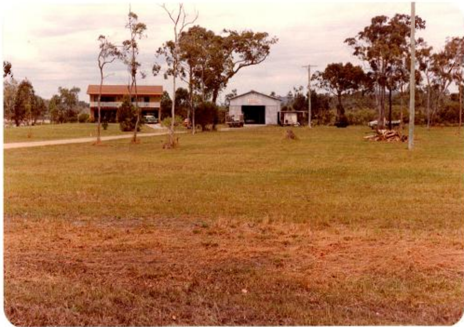
SITE OF AREA TO BE FILLED WITH SAND. NOTE HOW THE DWELLING IS CONSTRUCTED ON A MOUND. FILLING WILL BE PLACED TO WITHIN 100 M.M. BELOW THE FLOOR LEVEL OF THE DWELLING.
