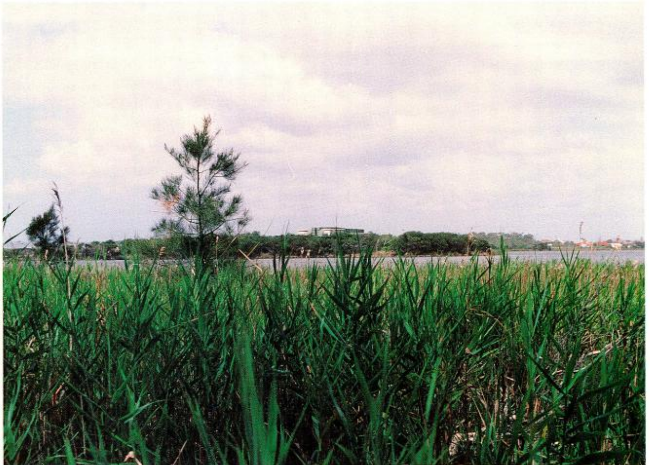
PLATE 3: VIEW OF JOHN DARLING NO. 4 VENTILATION SHAFT IN BELMONT LAGOON SHOWING THE HEIGHT OF THE FACILITY AND LANDSCAPING WHEN LOOKING TOWARDS THE SOUTHWEST.
