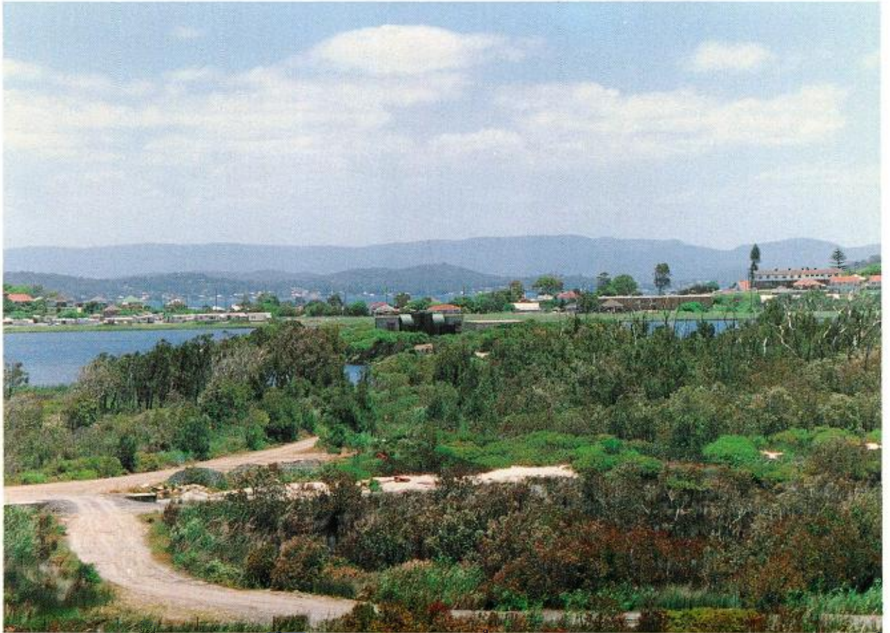
PLATE 2: GENERAL VIEW OF JOHN DARLING NO. 4 VENTILATION SHAFT IN BELMONT LAGOON, SHOWING THE AREA OCCUPIED BY THE FACILITY AND ITS SURROUNDS WHEN LOOKING TOWARDS THE WEST.
