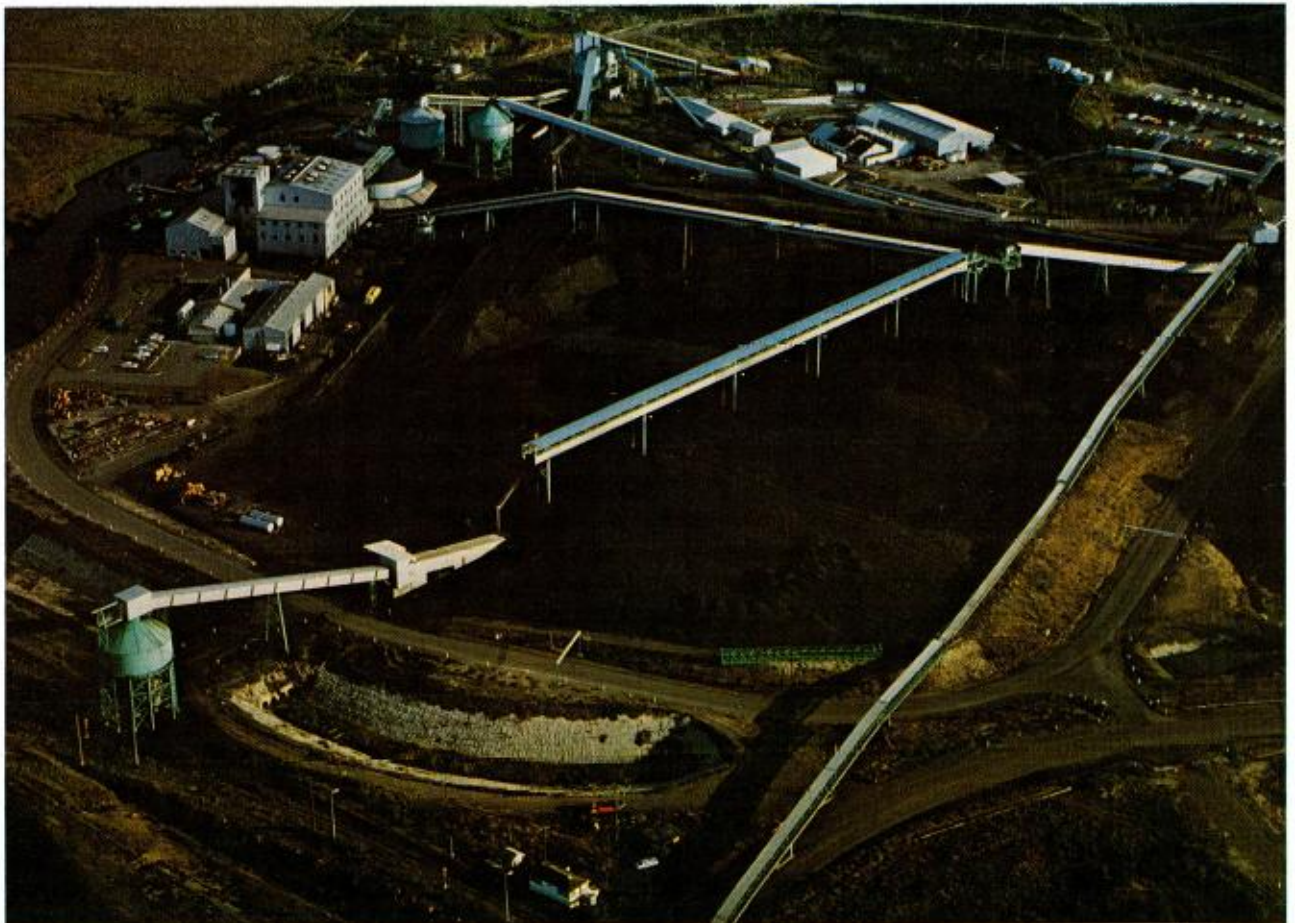
PLATE 7 LIDDELL COAL PREPARATION PLANT
