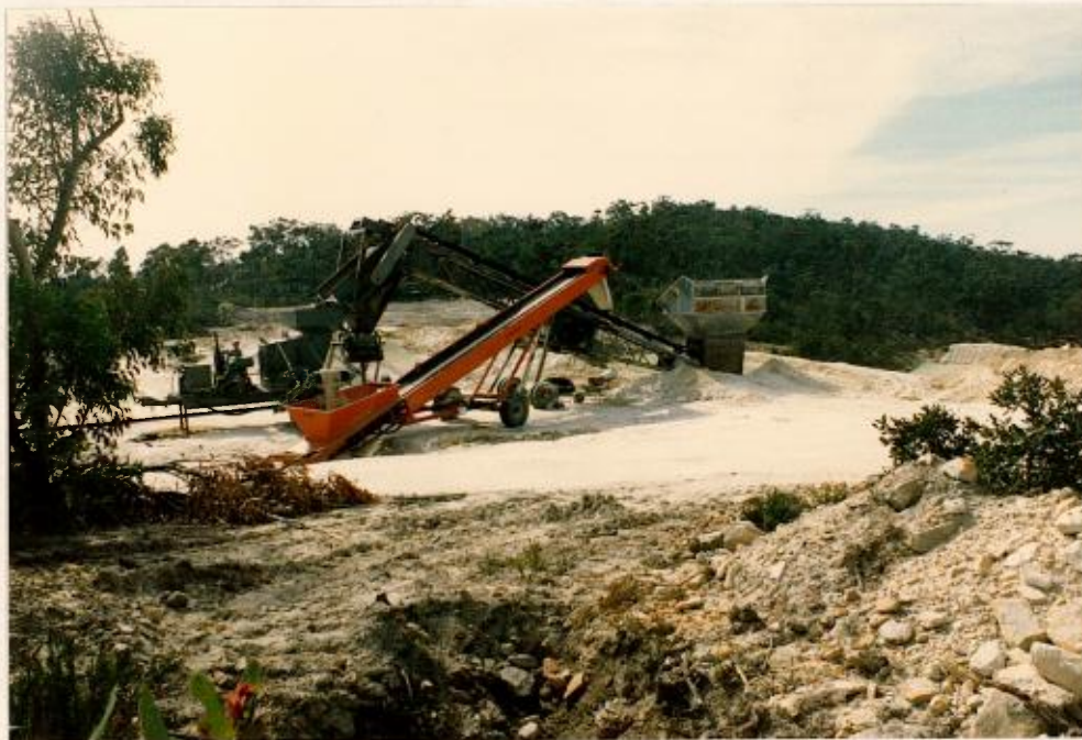
PHOTOGRAPH 4 Looking east to the washing plant and processing area.
