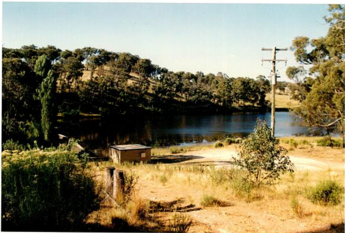
PLATE 6: A view to the north across Burraga Dam. The pump house is in the foreground. (Ref: 93/10)
