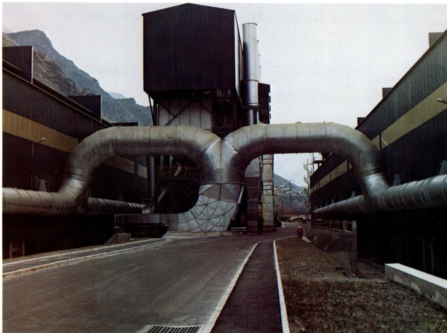
PLATE 5 DRY SCRUBBER AT THE ST JEAN de MAURIENNE SMELTER, FRANCE
