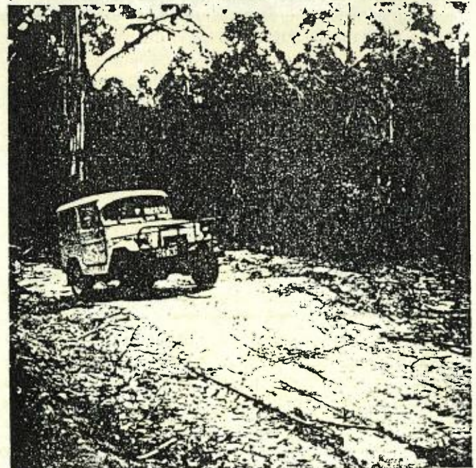
Figure 4. The bank of earth resulting from the spillway clearing can be left to act as a silt trap and water spreader.
