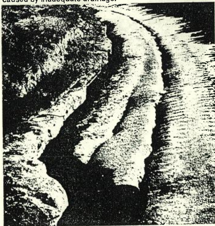
Above: Trafficability is seriously impaired when undrained low standard roads become eroded. Below: Deep rill erosion caused by inadequate drainage.
