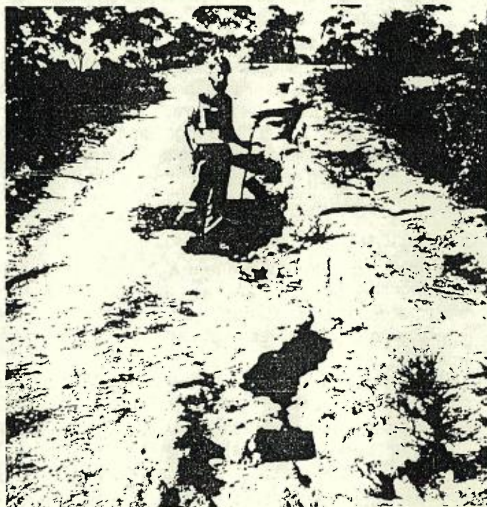
Above: Trafficability is seriously impaired when undrained low standard roads become eroded. Below: Deep rill erosion caused by inadequate drainage.
