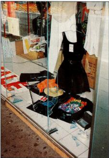
35. Window glass broke in several shop fronts in Hunter Street during the earthquake. In other cases, rubber seals holding windows in place worked loose, necessitating removal of the glass in order to make repairs. (Photograph by courtesy of C. Featherstone)
