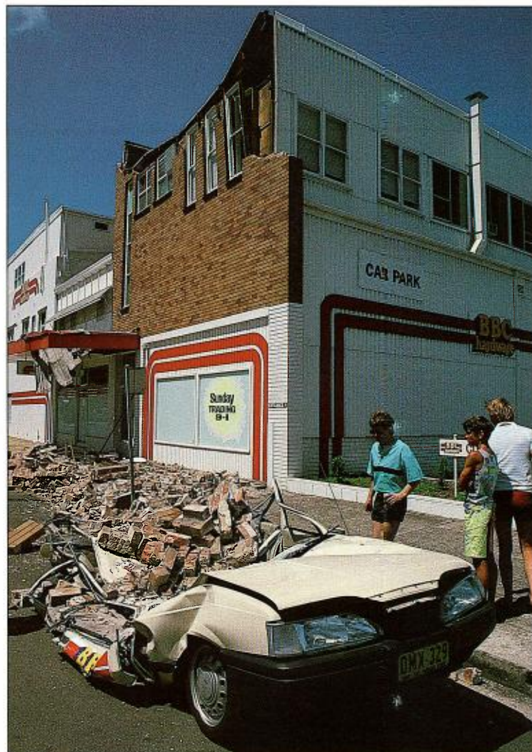
32. Ground motions are greatest at the tops of buildings. Parapets commonly fail because they are poorly supported, producing large amounts of debris in the streets. (Photograph by courtesy of K. Schreiber)
