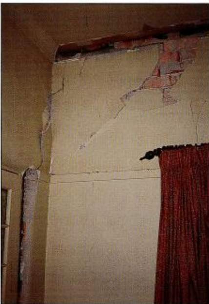
37. Numerous homes suffered minor damage. Typically unreinforced masonry walls moved, cracking plaster. Fallen cornices were a common form of damage. (Photograph by courtesy of C. Featherstone)
