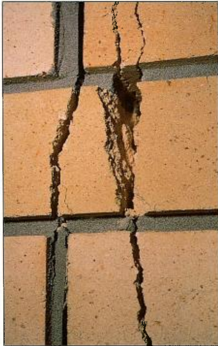
20. Close-up of damage to light-coloured modern bricks at Kotara High School constructed in 1968. These bricks are generally underfired to produce the light colour. (Photograph by courtesy of GIO (NSW))
