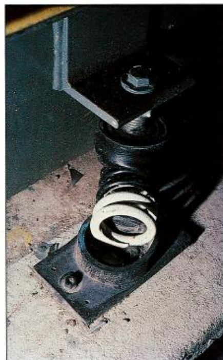
43. A typical displaced mounting. (Photograph by courtesy of the GIO (NSW))
