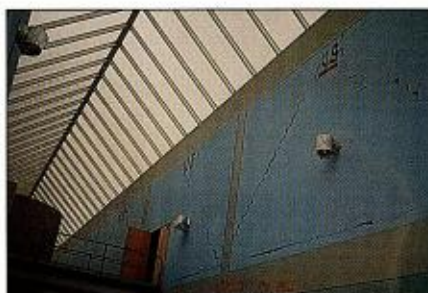
29. Brick in-fill panels at Rankin Park exhibit severe cracking typical of transverse wall failures. The reinforced concrete frame structure of the building was undamaged. "US" written on the walls means "unsafe". (Photograph by courtesy of C. Featherstone)
