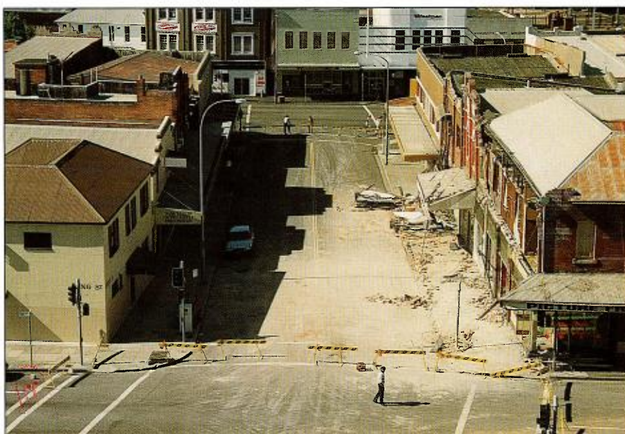
34. Road closures occurred in the Central Business District and in Beaumont Street, Hamilton because facades, awnings and parapets had fallen in some areas and because the structural safety of some buildings was suspect. Street closures, which lasted up to twelve days caused large losses on business interruption policies. (Photograph by courtesy of K. Schreiber)
