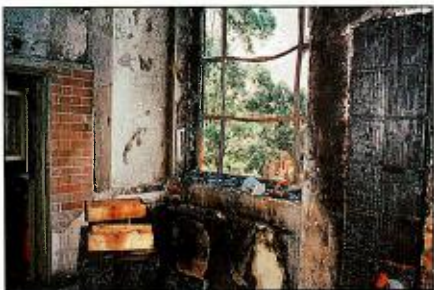
39. Damage resulting from a fire at Newcastle TAFE College. The fire occurred in a laboratory where chemicals were spilled by the ground shaking. This was the only reported example of fire resulting from the Newcastle Earthquake. (Photograph by courtesy of the GIO (NSW))
