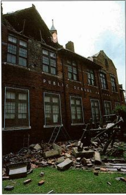
22, 23. The top of this wall at Wickham Public School leans outwards by 7-10 cm. The gable on the front of the building has also been damaged producing large amounts of debris in the school playground. If the earthquake had occurred on a normal school day many children may have been injured. (Photographs by courtesy of the GIO (NSW))
