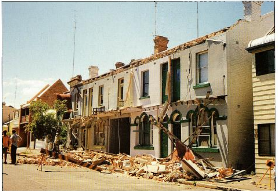
32. Ground motions are greatest at the tops of buildings. Parapets commonly fail because they are poorly supported, producing large amounts of debris in the streets. (Photograph by courtesy of K. Schreiber)
