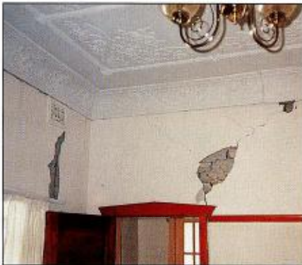
36. Cracking of brick and plasterwork in a typical older unreinforced masonry residence in the suburb of Merewether. While often not serious, such damage can be expensive to repair. (Photograph by courtesy of C. Featherstone)
