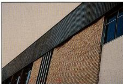
28. Wall failure at the Hamilton R.S.L. Club, a steel-framed building with brick in-fill panels. After the earthquake it was possible to push bricks out from the inside by hand. (Photograph by courtesy of C. Featherstone)
