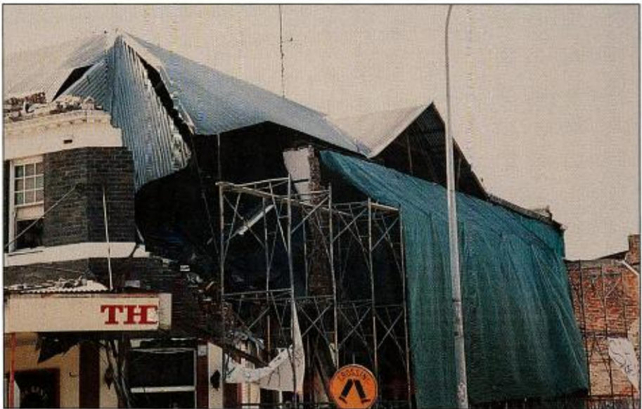
27. The gable end, parapet and front wall of the Kent Hotel in Beaumont Street, Hamilton fell into the street, demolishing the awning and killing two people. (Photograph by courtesy of C. Featherstone)
