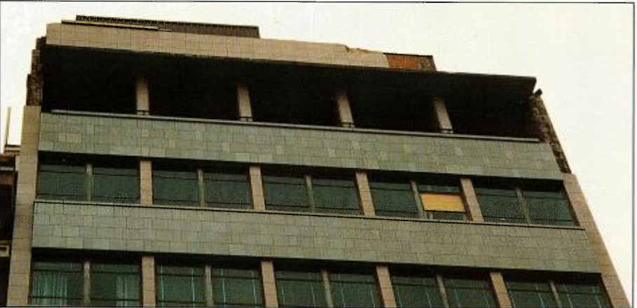
19. The QBE Insurance building. This modern high rise reinforced structure suffered damage to the top floor and part of the parapet, emphasising that damage is concentrated at the top of the building. (Photograph by courtesy of C. Featherstone)
