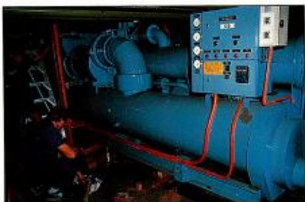
40. This airconditioning unit, on the top floor of a modern building moved off its mounting during the earthquake. The workmen are using hydraulic jacks to move the unit back into position. (Photograph by courtesy of C. Featherstone)
