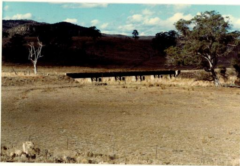
Figure 27(10) Wollar Creek Bridge (Bridge No. 10)
