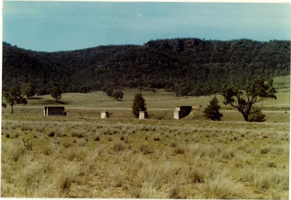
Figure 6. Typical bridge on existing railway formation.
