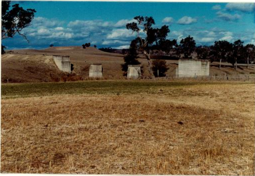
Figure 27(9) No. 3 Goulburn River Crossing (Bridge No. 9)
