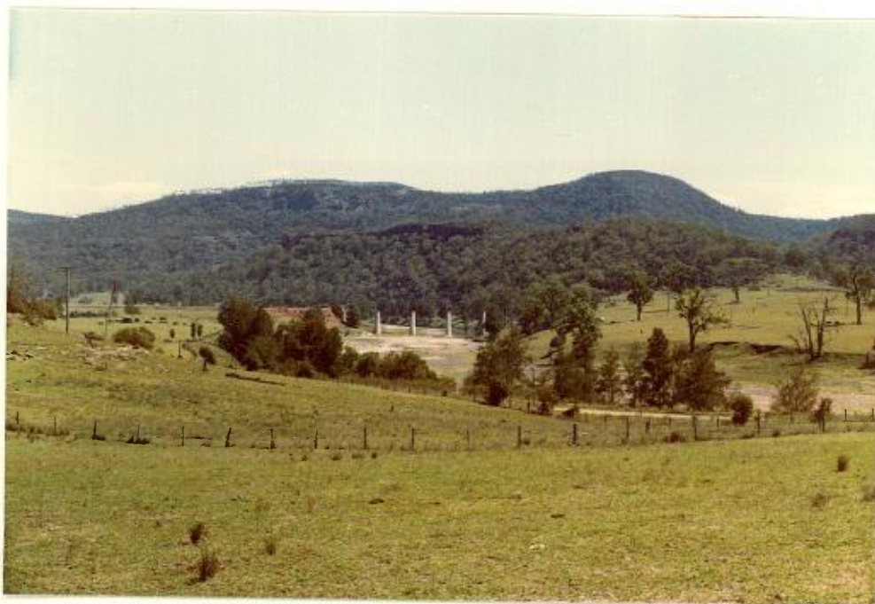
Figure 27(8) No. 2 Goulburn River Crossing (Bridge No. 8)
