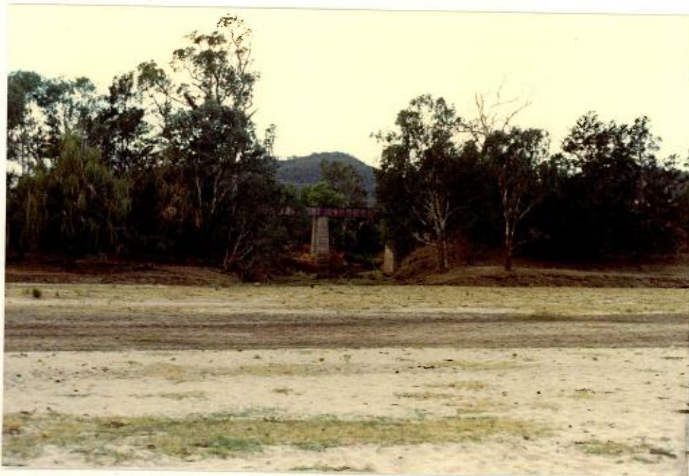
Figure 27(2) Worondi Rivulet Bridge (Bridge No. 2)
