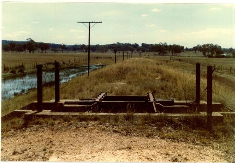
Figure 4. View along substantially complete railway formation.
