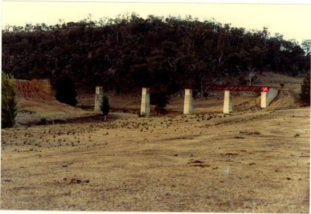
Figure 27(3) No. 1 Goulburn River Crossing (Bridge No. 3)
