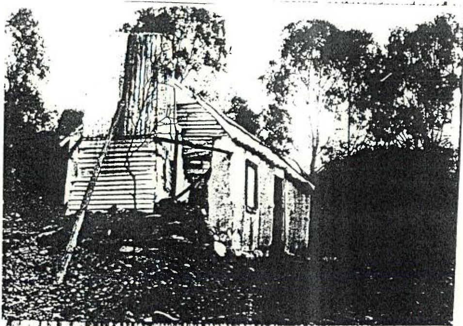
Figure 4.8: Privately built and owned housing at Newnes, note stacked stone around fireplace.
