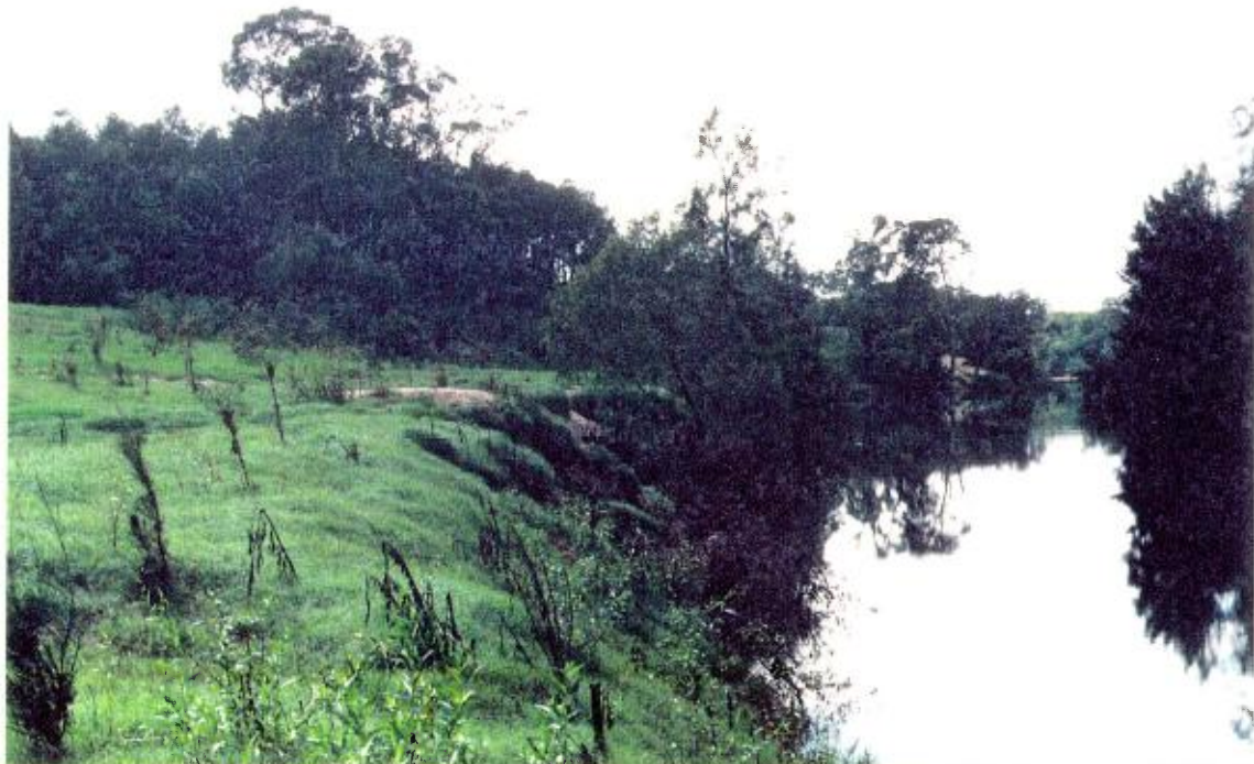
FIGURE 8 - Previously Extracted Soil Deposit Beside River on Spring Farm. View Upstream
