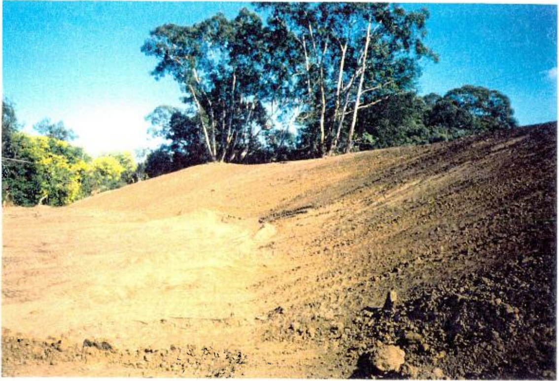
FIGURE 42 - Backfilling and Recontouring Extraction Area Ready for Rehabilitation
