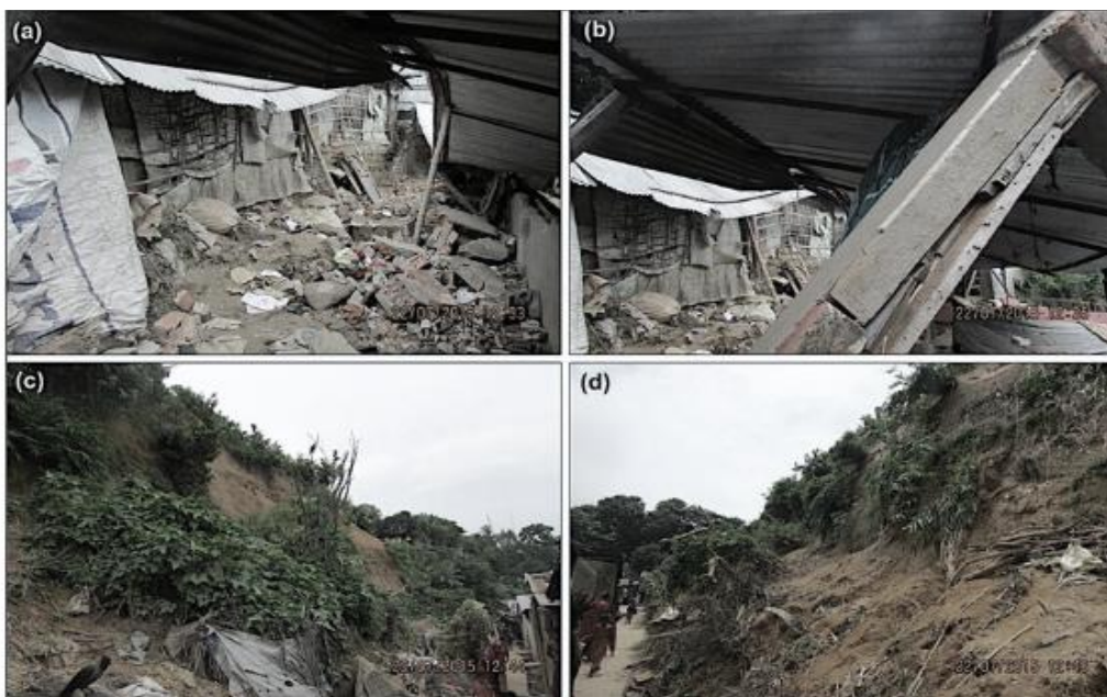
Figure 5: Devastation landslide on 19 July 2015 in Chittagong Metropolitan Area.
