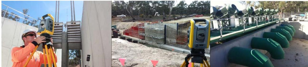
**Lock 15 Euston Weir and Fishway Upgrade:** High order set-out survey required for the Euston Lock and Fishway Upgrade sub-contracted to McConnell Dowell Contractors and pier raising and refurbishment. Survey tasks include control survey, horizontal and vertical survey control of new pier locations, as built surveys and verification plans deliverable to client in complex riverine environment.
