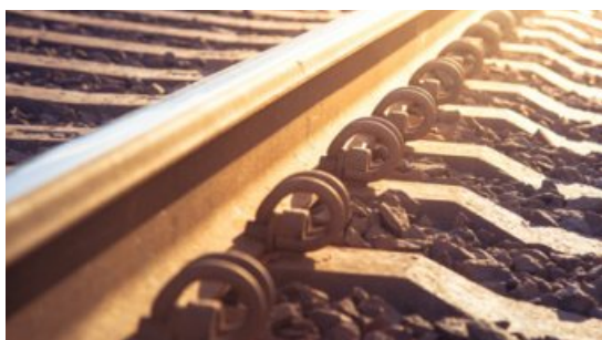
E-clip railway fastening system
