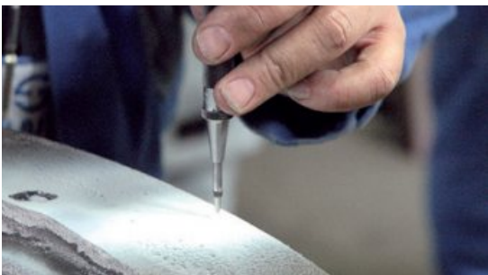
Drill position marking
