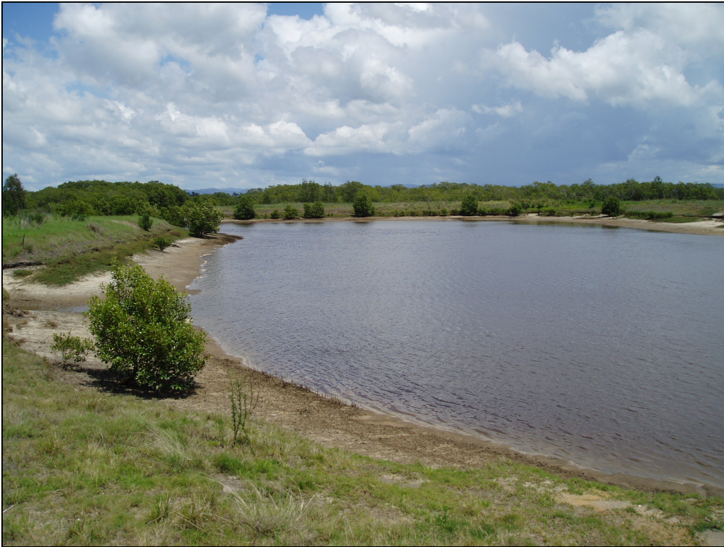
Plate 2. Large excavation in the centre of the A0S1 unit; the spoil will now contain activated ASS
