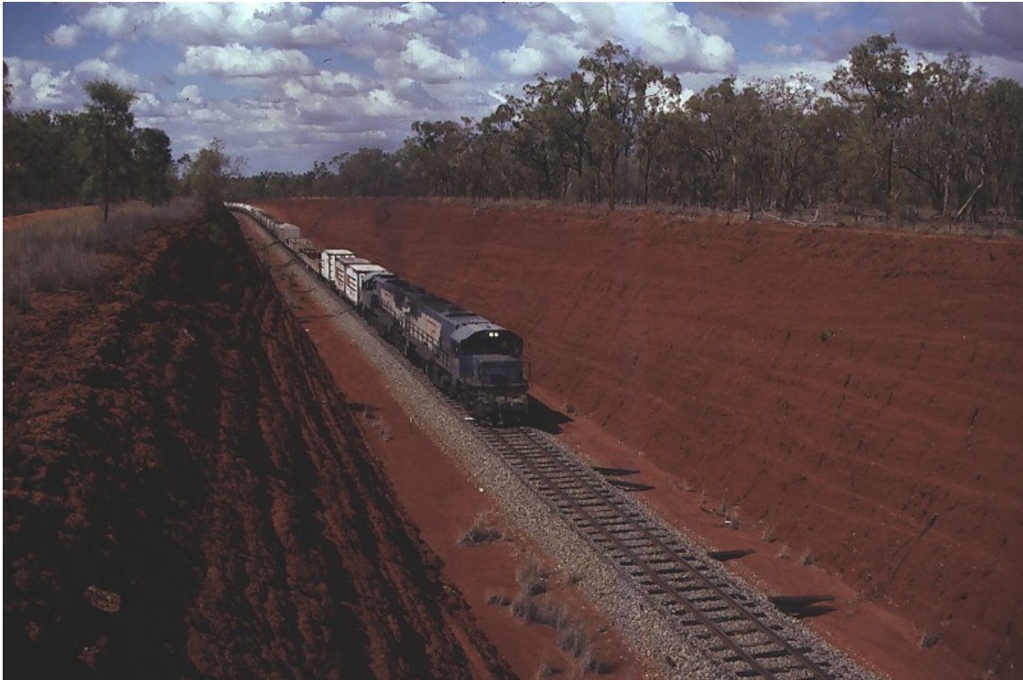
Figure 3.6 A railway cutting near Pentland provides a good depth indicator for the sandy Red Kandosols on the sandsheet that characterises the Desert (DT) and Grant (GT) land systems extending south to Barcaldine
