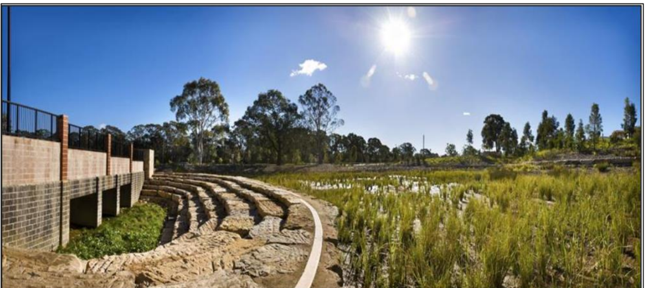
Figure 6-1 Example of Urban Bio-Retention Basin (Courtesy Water by Design)
