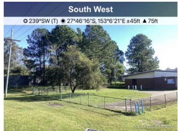
Plate 6: Existing community infrastructure building, adjacent to site
