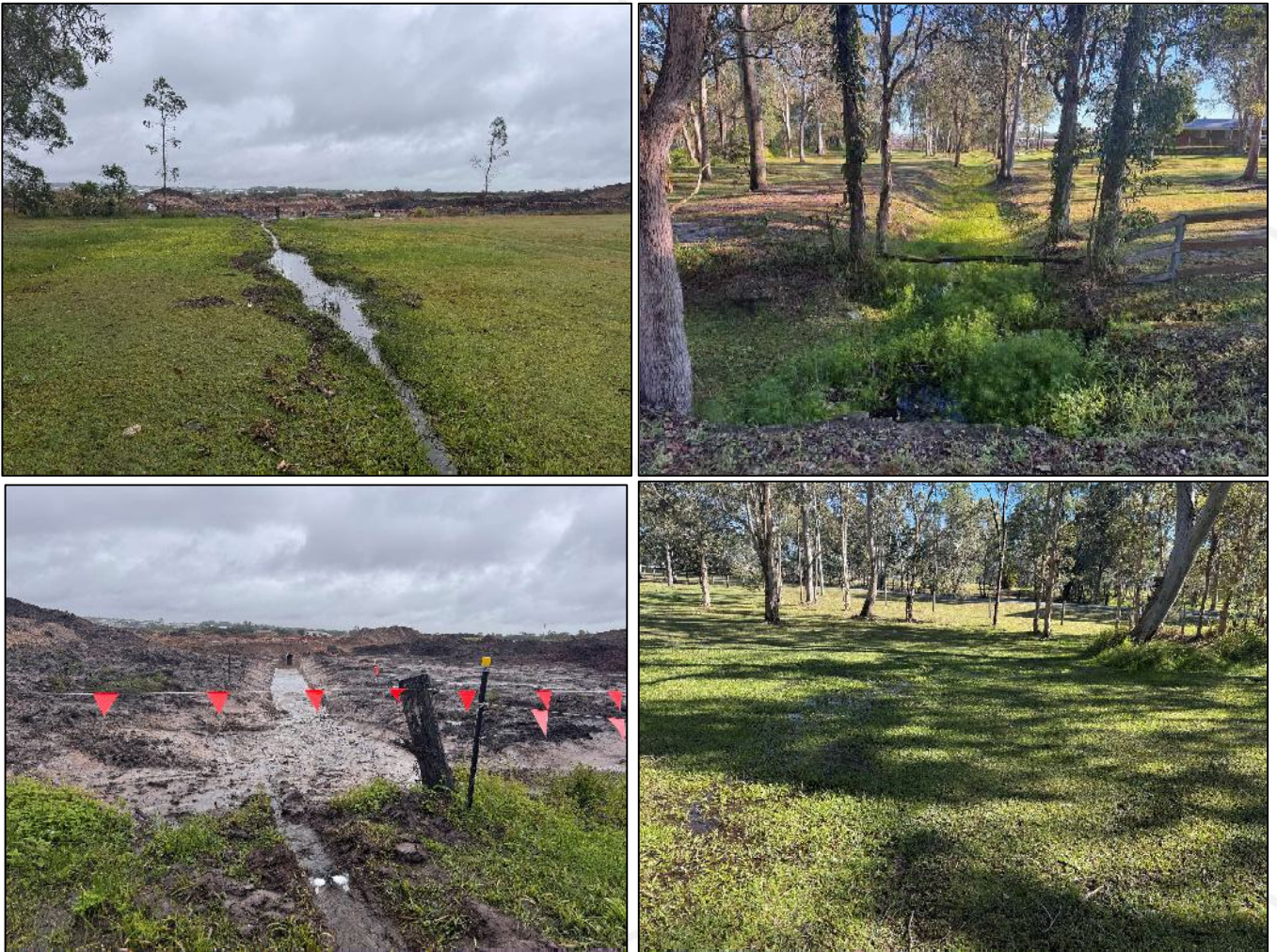
Photo set 1: Pooling water present on Lot 801 (top left), native water tolerant vegetation on Lot 801 leading to the Calume Court culvert (top right), development adjacent to the northern boundary of Lot 801 (bottom left) and overland flow path with maintained lawn on Lot 15 (bottom right).
