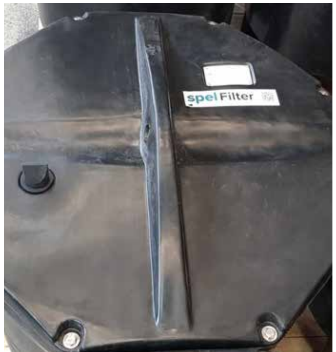
Figure 6 - the top of the SPELFilter showing the location of the one way air valve
