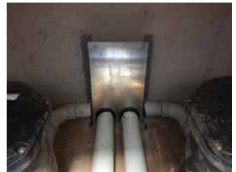
Figure 3 - Typical Outlet Weir Wall
