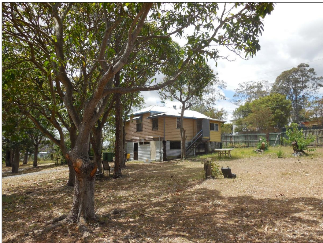
Photo 2: Existing Uninhabitable High-set Houses at the Subject Site (to be demolished)
