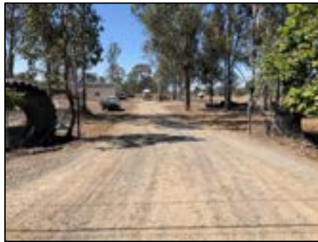
Access Driveway leading into the Property
