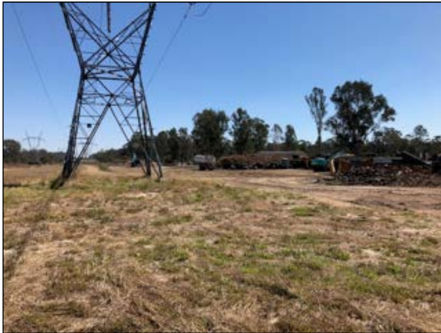
Vegetation beneath transmission Lines passing through the property
