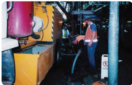
Photo 11 Cleaning an EnviroPod using the inductor method
