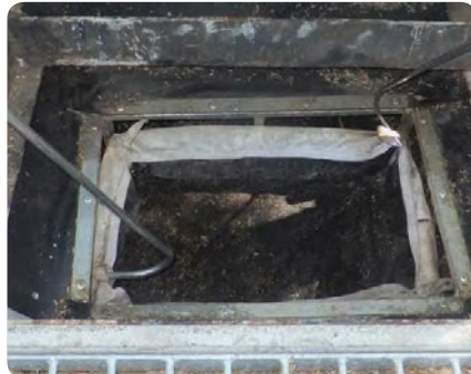
Photo 21 Correctly installed filter bag
