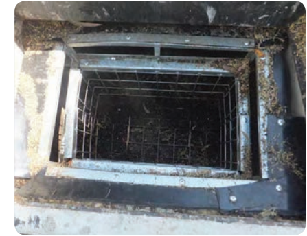
Photo 24 Check joining rivets (two piece unit shown above)
