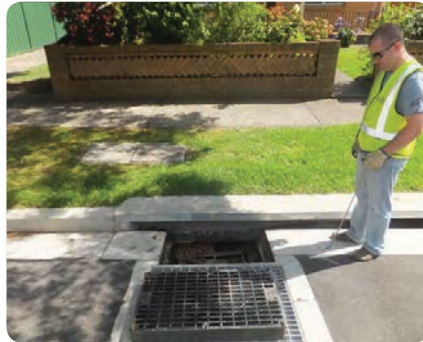
Photo 4 Fully open grate
