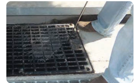
Photo 6 Insert hook near edge of grate
