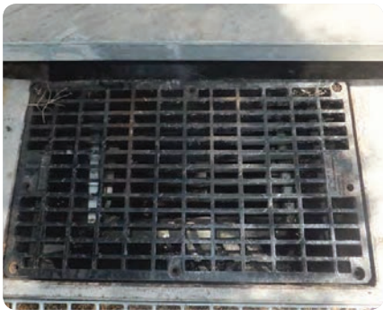
Photo 22 Installed filter bag and sealed pit
