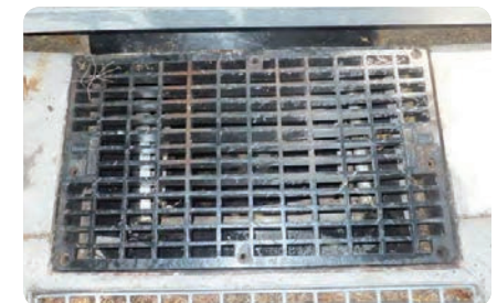
Photo 10 Reinstated non hinged grate
