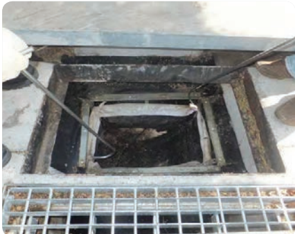
Photo 20 Ensure that the unit is positioned correctly, with the lifting loops on the inside
