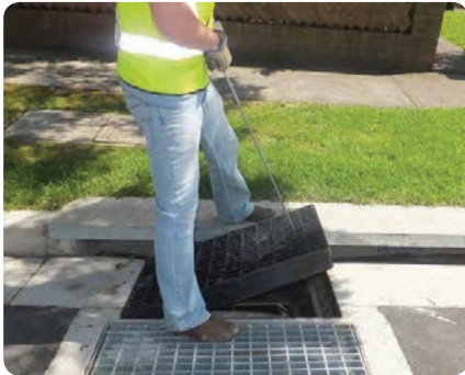
Photo 3 Lifting the grate
