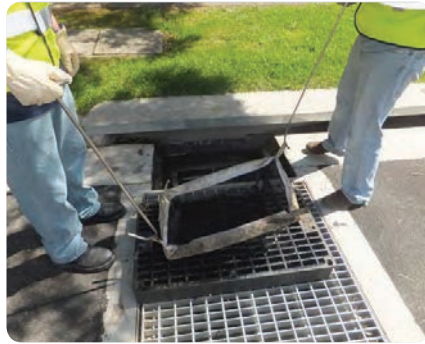
Photo 19 Reinstall filter bag
