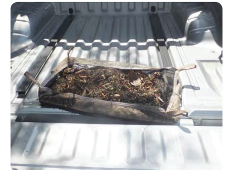
Photo 15 Lift the bag onto the collection vehicle
