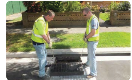
Photo 8 Lift grate and move grate to one side
