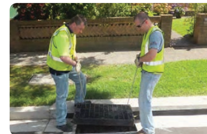
Photo 9 Lift grate above the support frame
