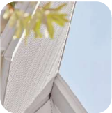
COLORBOND ROOF SHEETING
