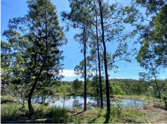
Plate 11 View facing northwest of dam.
