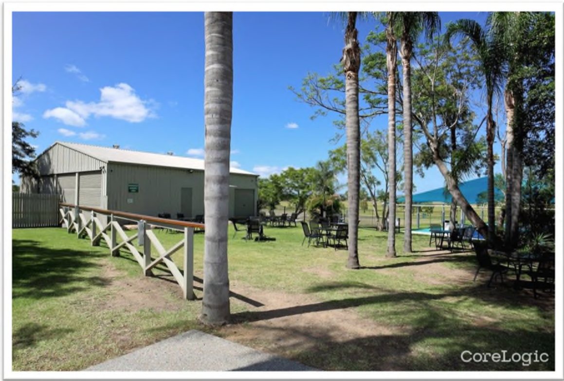
Site Photo 4: View towards the existing building proposed to be converted to a shop (source: RP Data)
