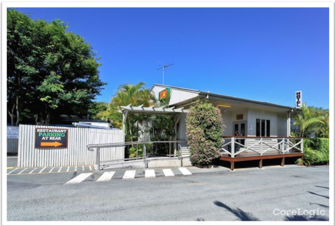
Site Photo 2: View of the existing hotel building from within the Subject site (source: RP Data)
