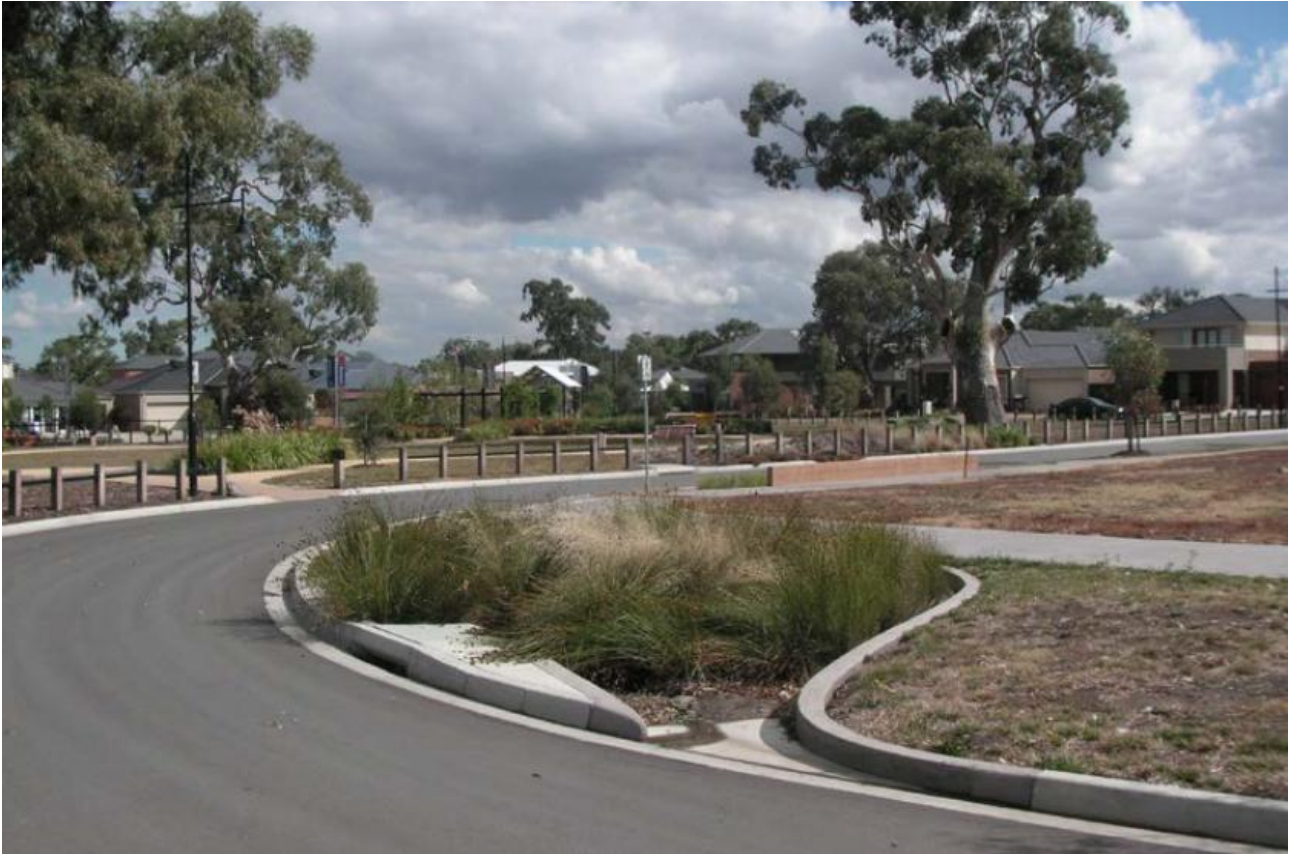
Figure 7-2 Example of a WSUD Bio-Retention Verge Pod Design (Image Courtesy: Water by Design)
