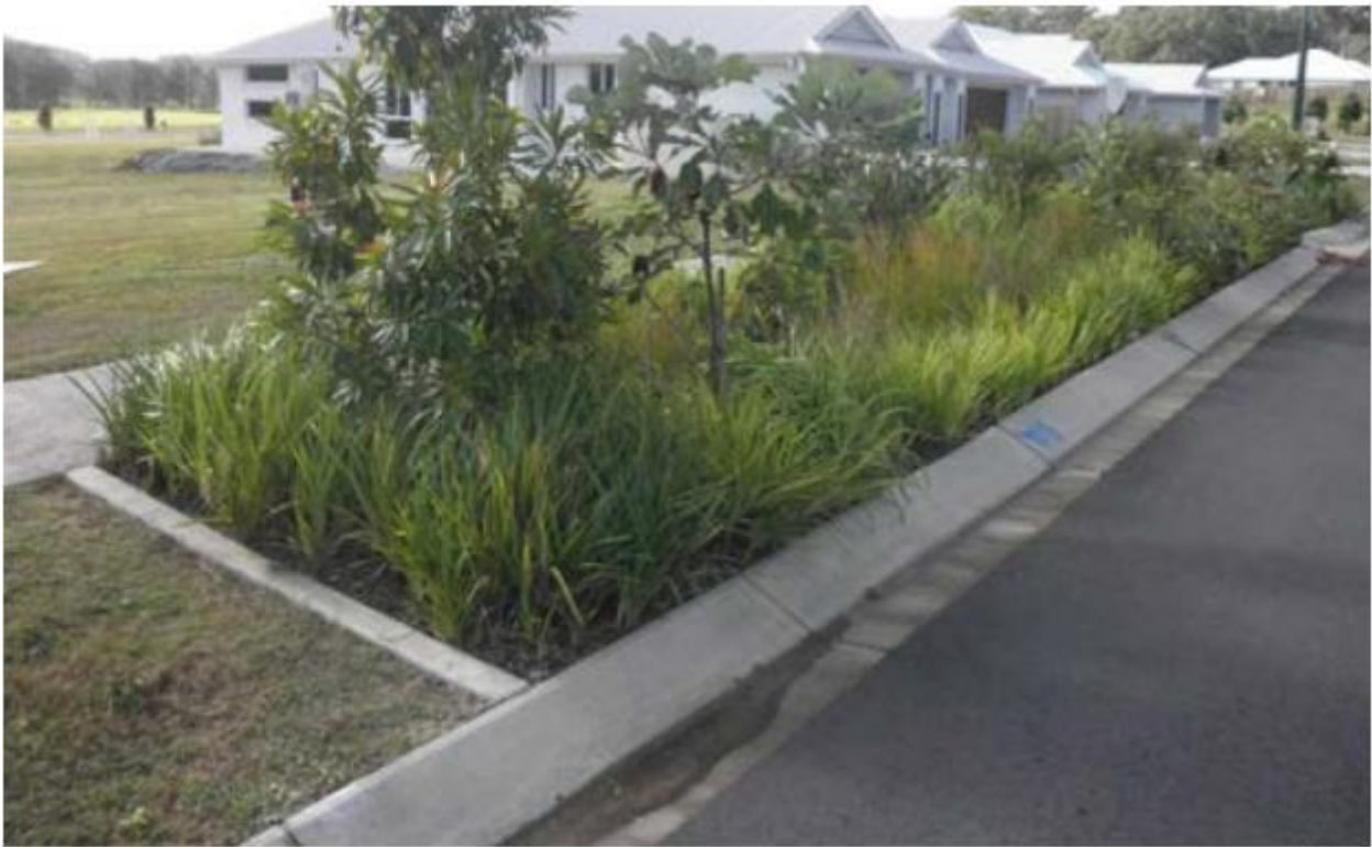
Figure 7-1 Example of a WSUD Bio-Retention Verge Pod Design (Image Courtesy: Water by Design)
