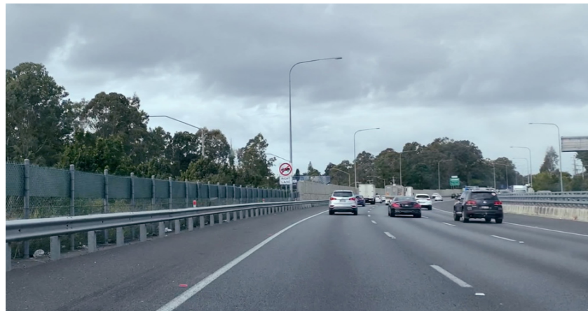
EXISTING SOUTHBOUND VIEW DISTANT
