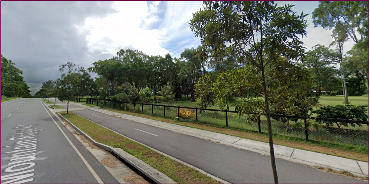
Figure 4 – Existing Streetview from Mountain Ridge Road
