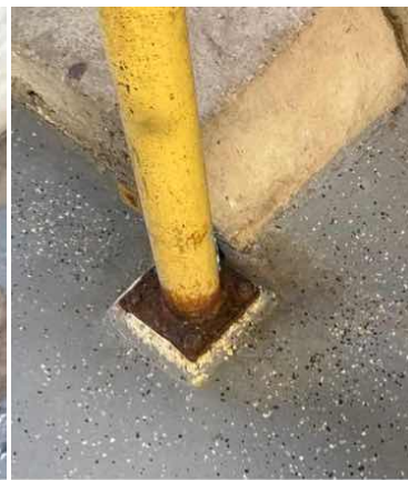
Example of corroded posts
