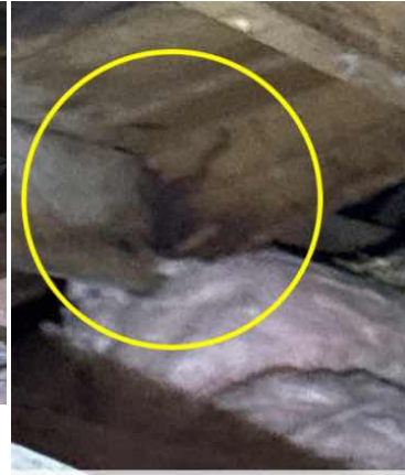
Example of evidence of leaking, photo from above the family / meals
