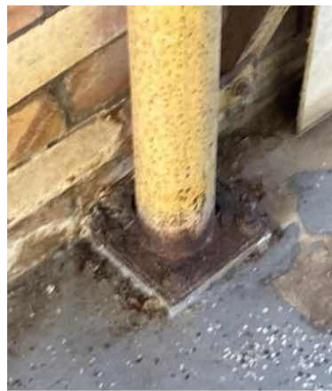
Example of corroded posts
