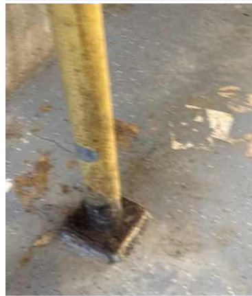
Example of corroded posts
