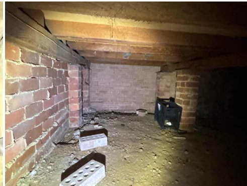
Formwork remains beneath the entry porch
