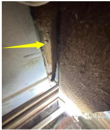
Sole plates with decay and termite workings, photo beneath the bathroom
