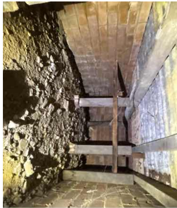
Formwork remains beneath the entry porch
