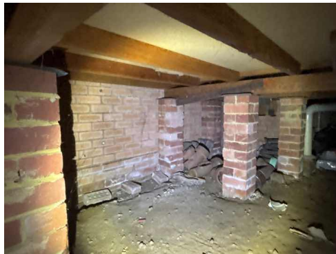
Formwork remains beneath the entry porch
