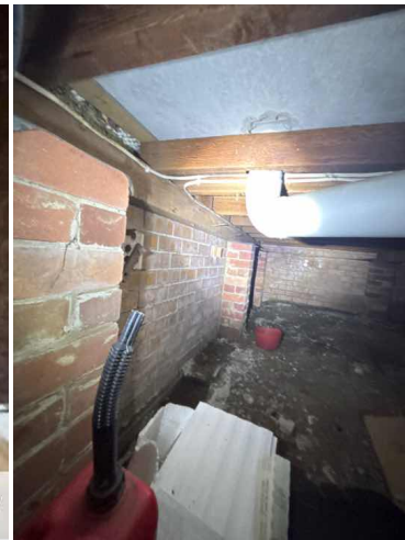
Sole plates with decay and termite workings, photo beneath the bathroom
