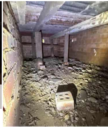
Formwork remains beneath the entry porch
