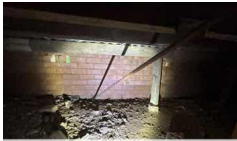
Formwork remains beneath the entry porch
