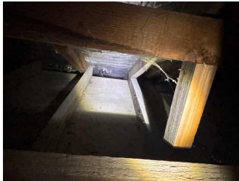
Example of termite workings in top plates, photo from above the bathroom
