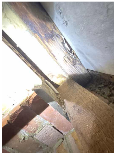
Sole plates with decay and termite workings, photo beneath the bathroom
