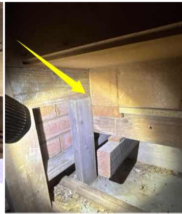
Example of termite workings in stairs adjacent to the bathroom
