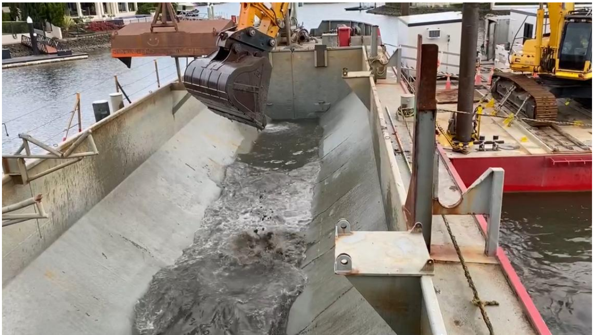
Plate 1. Example images of spud barge with excavator loading a self-propelled split hopper barge.
