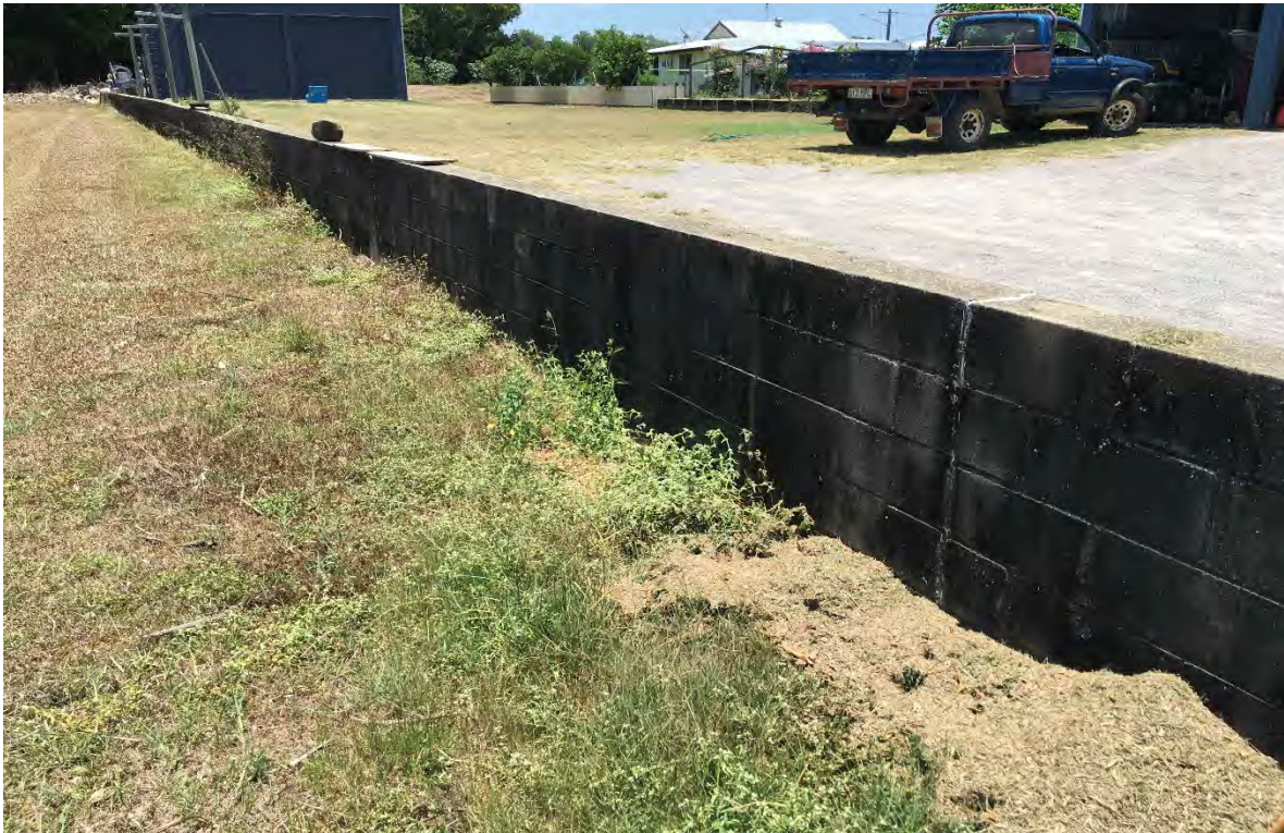
Halifax Levee. Concrete block section in the residential area
