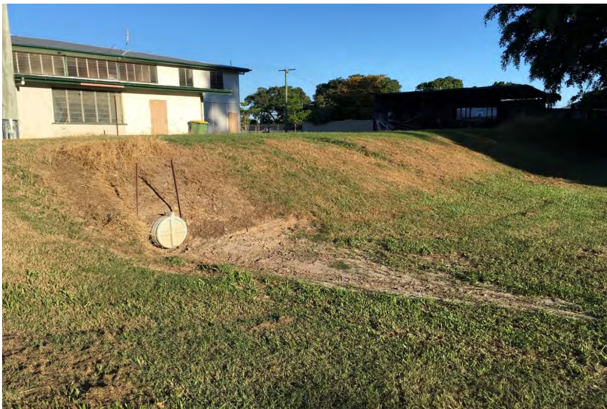
Halifax Levee. Earth section in the business area. Floodgate to clear local drainage
