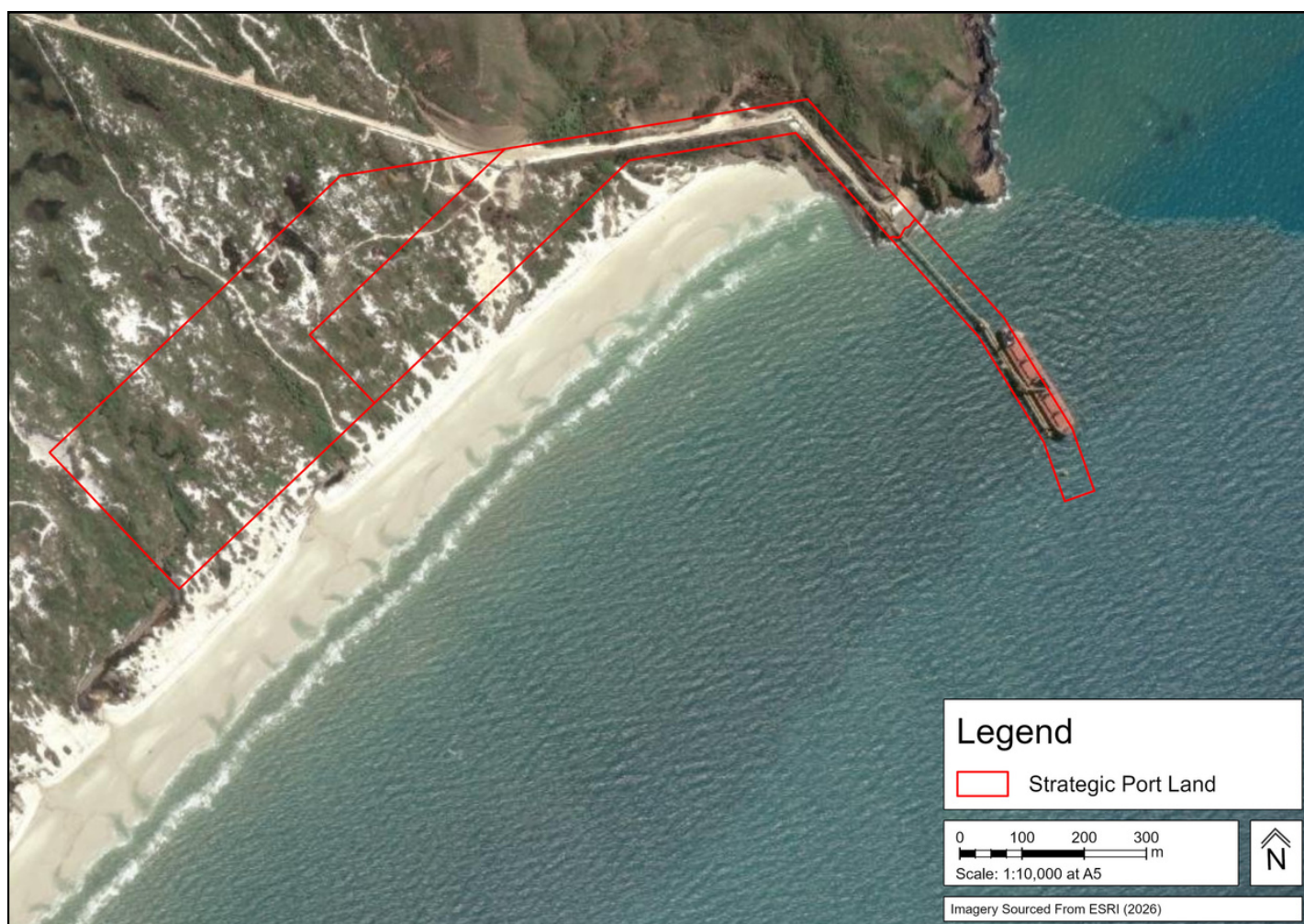
Figure 1 - Aerial Photograph – Strategic Port Land
