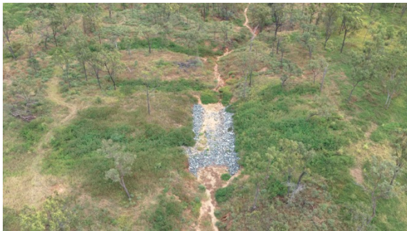
Figure 3 Rock Shutes post construction and post wet season
