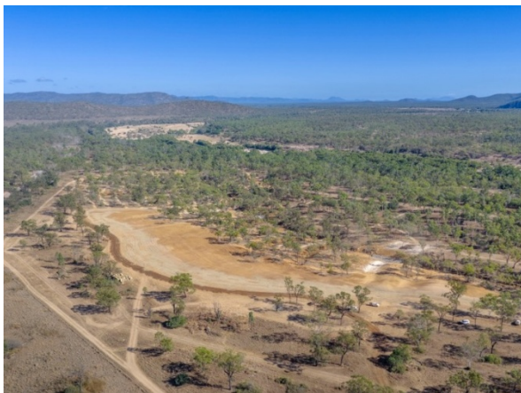
Figure 1 Post work -October 2025
