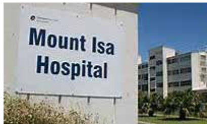
Key System upgrade for Queensland Health North West Region
