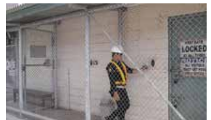
Fencing and Access Readers for Process Plant in Gosowong, Indonesia
