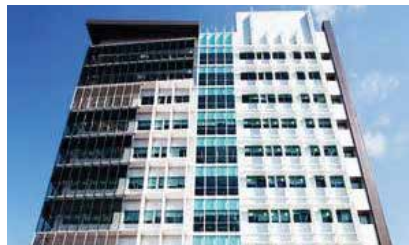
Verde Townsville Electronic Security with Door Hardware and Key System
