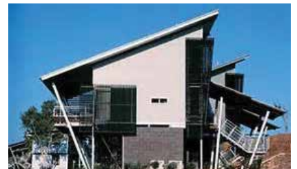
Door Hardware and Key System upgrade for Lavarack Barrack JLU
