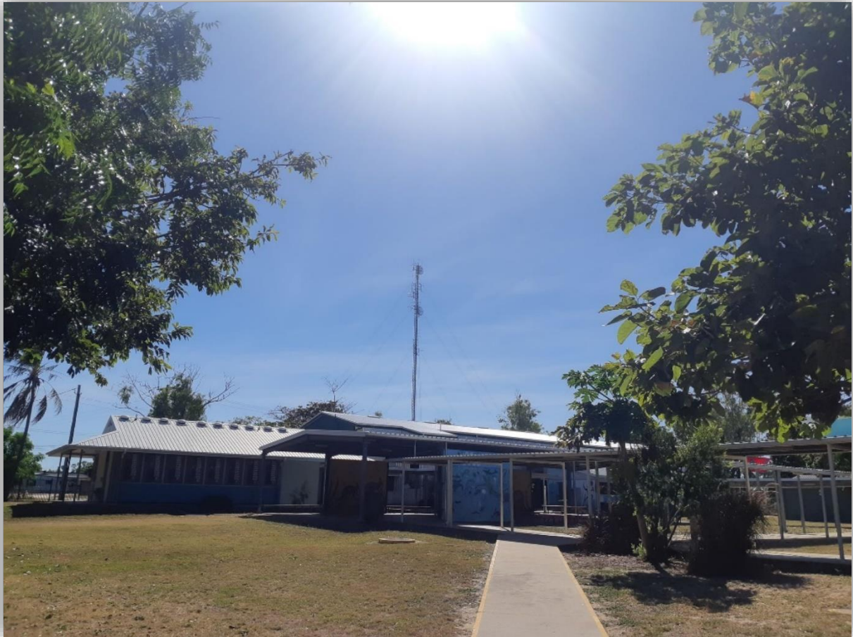
Pompokuraaw State School and Communication Tower
