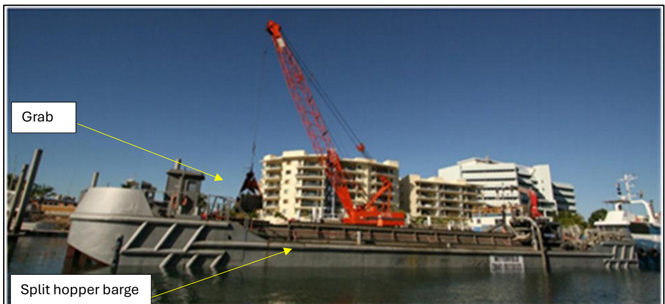
Figure 42: Mechanical Grab Dredge and Split Hopper Barge.
