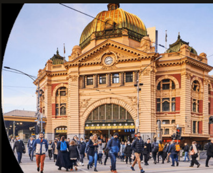
FLINDERS ST STATION · OPPOSITE
