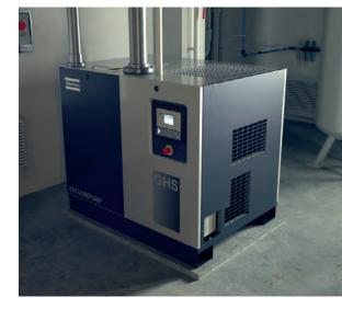
Due to its plug-and-play design, the series assures an easy and fast installation that saves time and space. The footprint is no larger than that of a standard pallet and everything required is delivered as a complete package.
