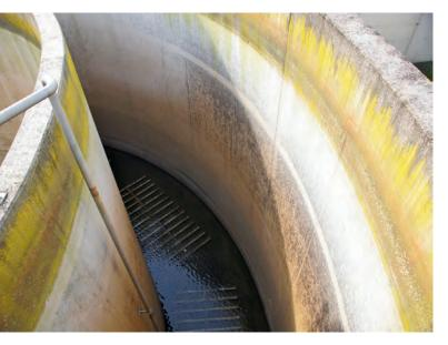
"The biological process takes place in eight tanks that are subdivided into four lines," explained sewage water technician Reinhard Schweinforth. The tanks are 10 m high with a water depth of 8.5 m - unusual dimensions for sewage treatment plants, noted Schweinforth, which are normally 4 to 5 m deep. The air required for the biological cleaning process is blown
