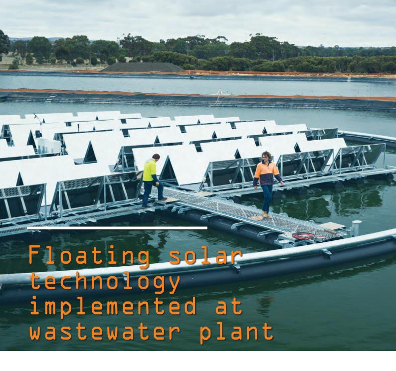
Infratech Industries has launched a floating solar system that will generate an estimated 57% more power than fixed land-based systems. he technology uses water to counteract the gradual loss of output caused by overheating solar panels to create a more efficient system.
