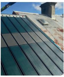
BlueScope Steel's project integrates solar PV modules into the roofs of homes.
