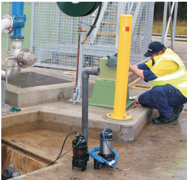
Barry Cook, Sydney Water, installs a TM series titanium pump at the sewage collection station at Douglas Park to handle the sewage spills during transfer to collection tankers.
