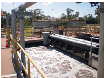
Diffusers in action at South Rockhampton Sewage Treatment Plant providing high-efficiency oxygen transfer and generous mixing.
