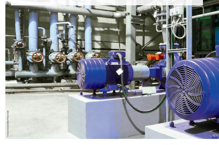
n the quest to improve the energy efficiency of drive systems, much effort has been spent on improving the efficiency of the electric motor. Through the introduction of a classification system for motor energy efficiency in the IEC 60034-30 standard, users are given a clear and easy framework for comparing motor efficiencies.
