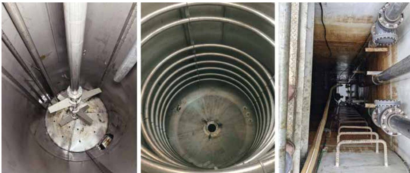
Figure 1: Equipment such as agitators, heating coils, pipes, ladders or baffles inside tanks can potentially interfere with microwaves and impact level measurement.
