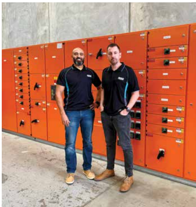
Progress Switchboards Sales Director Jay Wright, left, with General Manager Conor O'Shea, right.
