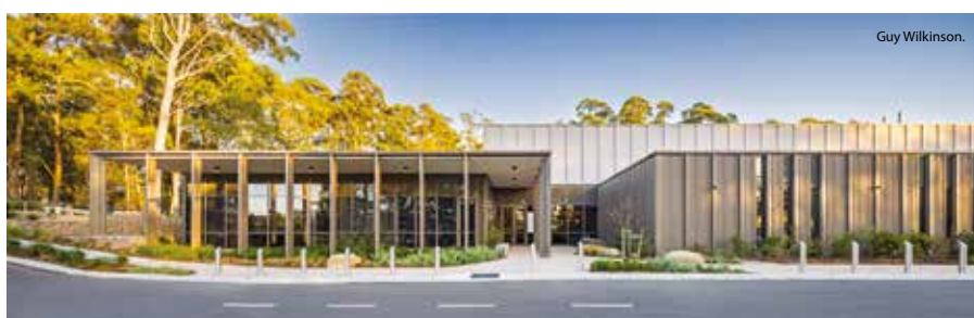
Above: Grounded within the surrounding eucalypt landscape, the RNA facility is designed to establish a calm civic entry that balances advanced manufacturing precision with warmth, shadow and a strong sense of place.
