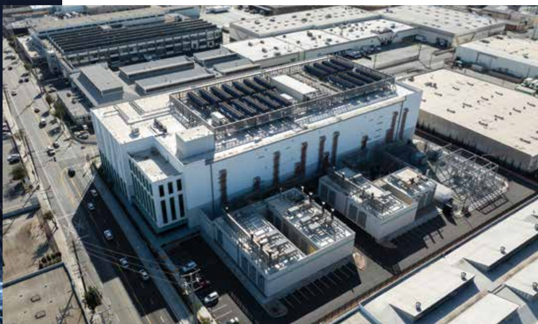
Data centre facility in Vernon, California, USA.
