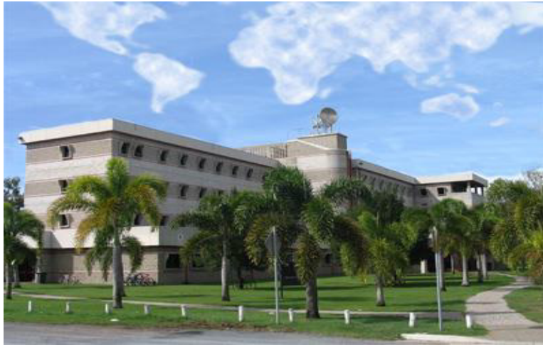
Figure. 1. Building no 19; at Rockhampton Campus of CQUniversity.
