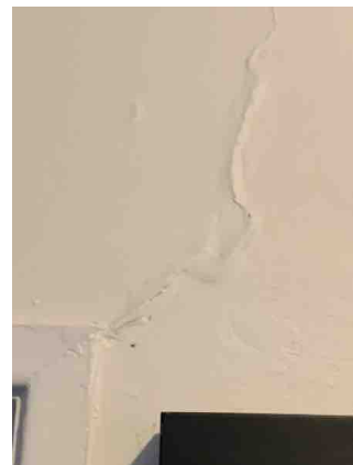
Wall cracking.
