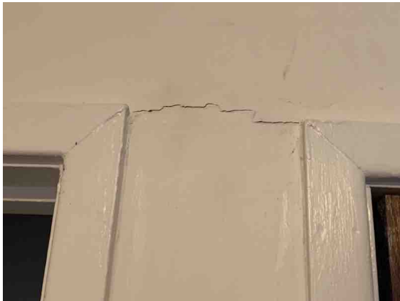
Horizontal wall cracking.
