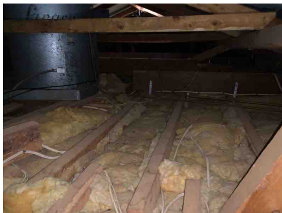
Insulation in the roof void area.
