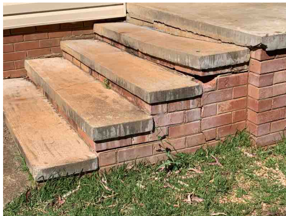
The verandah steps have moved and are damaged.
