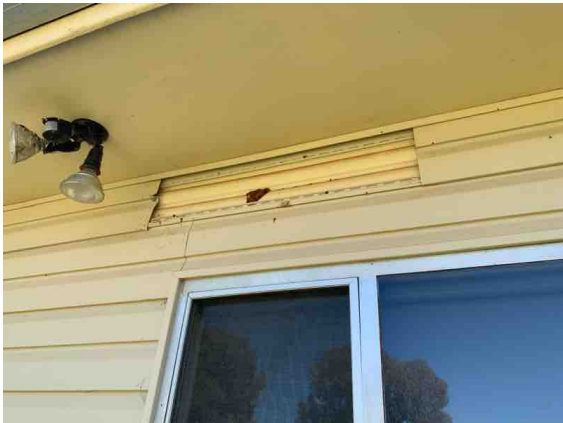
The damaged wall cladding.
