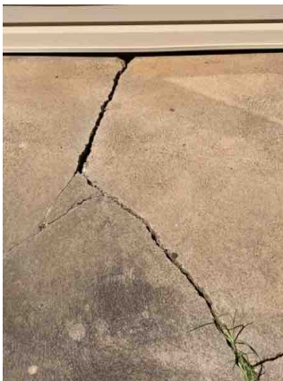
The cracked and failed concrete.
