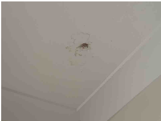
Water damaged ceiling sheeting.
