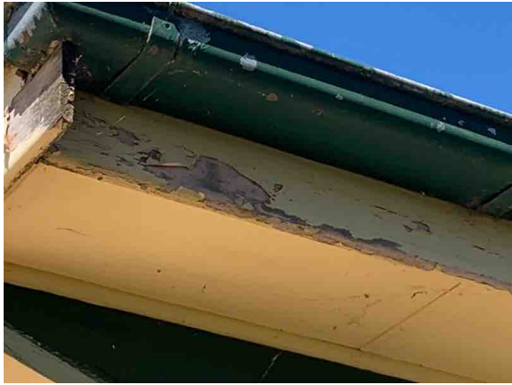
The deteriorating paintwork and timber.
