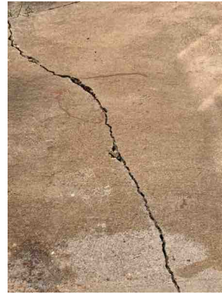
The cracked and failed concrete.
