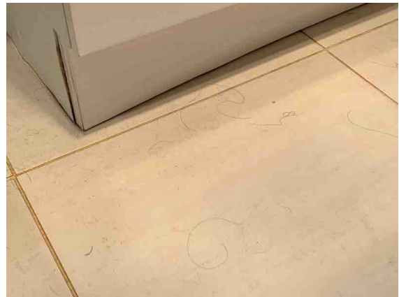
The water damaged vanity kick board.
