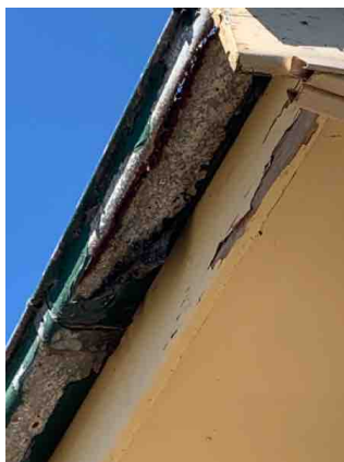
The damaged gutter.
