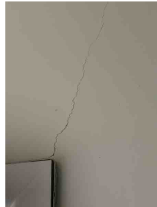
Wall cracking.
