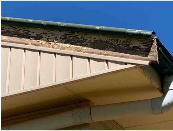
The deteriorating paintwork and timber.
