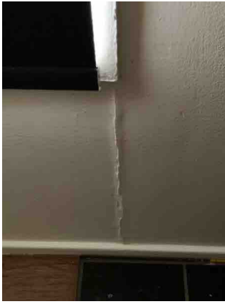
Vertical wall cracking.
