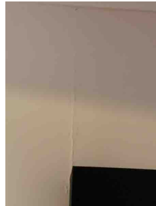
Vertical wall cracking.
